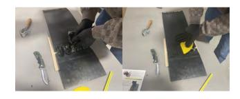
With clip joints, ensure that the FR1510 penetrates through all gaps between the pin and hinges. use spatula or putty knife.
